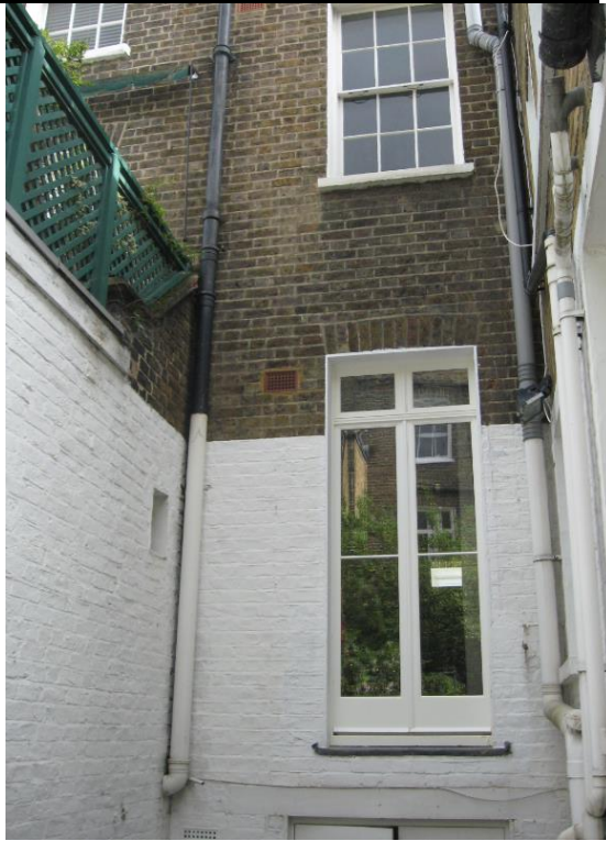
Rear Elevation (Prior to Works on the Basement Commencing)
